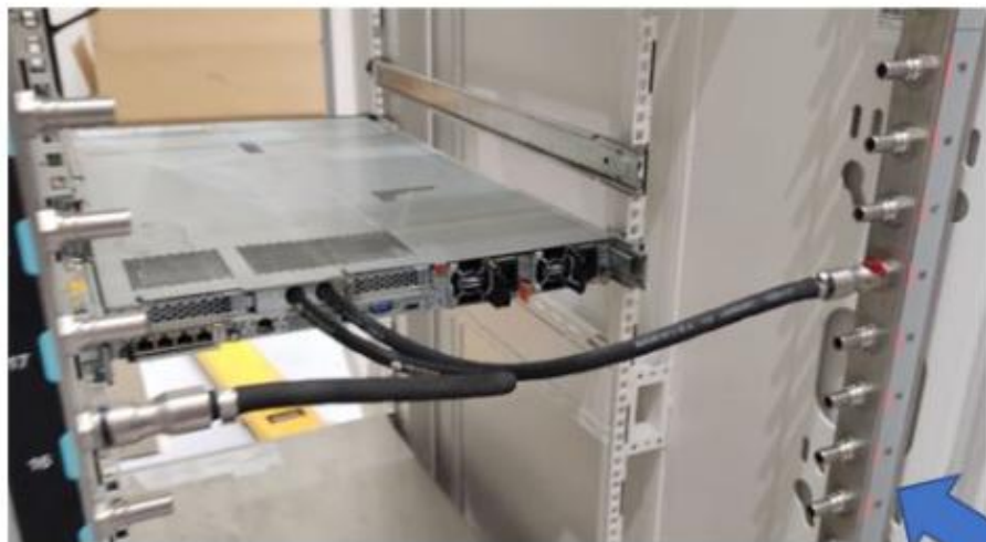
ThinkSystem Neptune DWC 38 Port Rack Manifold (inlet, outlet)
