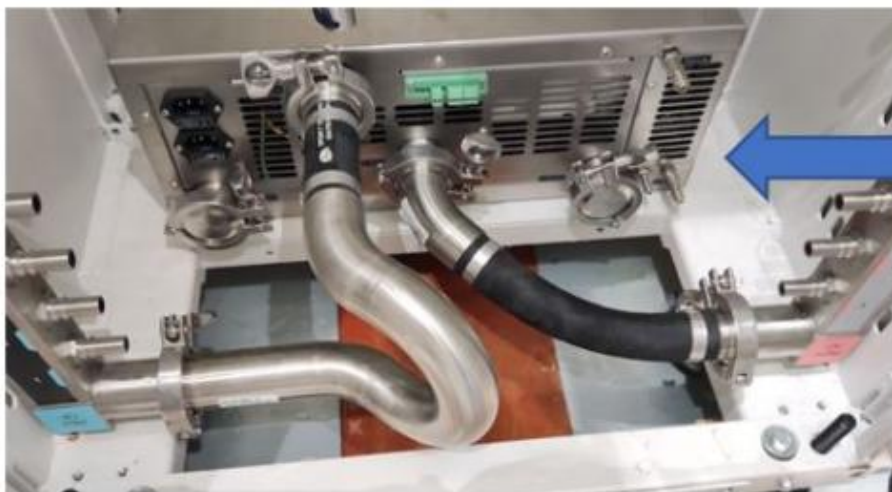
RM100 in-rack Coolant Distribution Unit (CDU)
